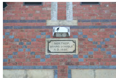
Patterned brickwork on the front
