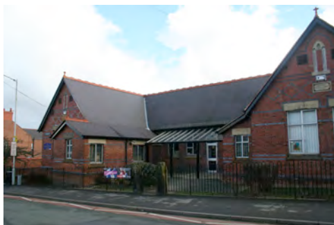
The 1881 part on Mold Road
